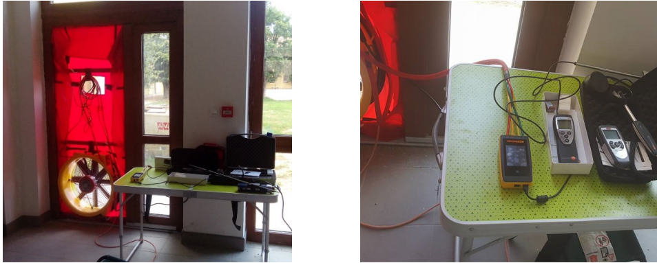
Figura 5.57 - Blower-door test set-up
