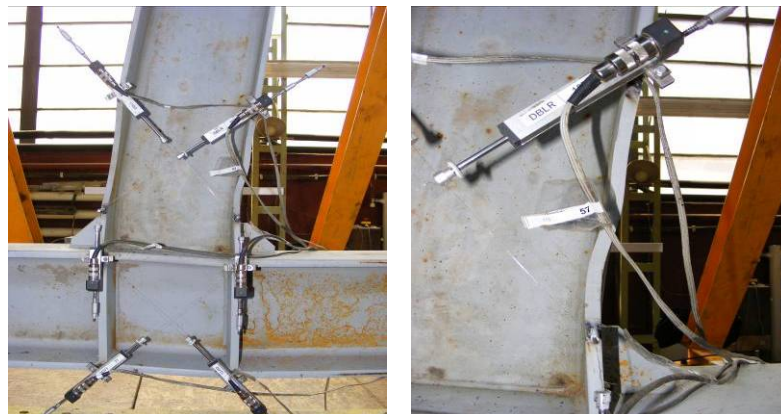
Fig. 3.64. Failure of the node with RBS at maximum displacement
