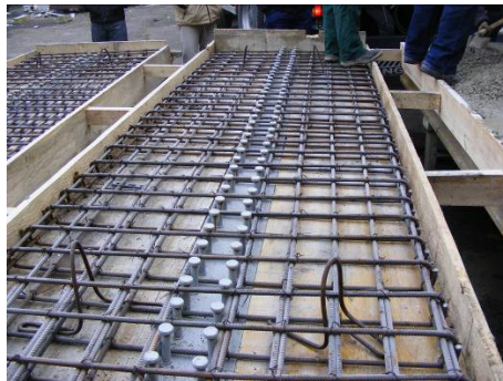
Fig. 3.22. Reinforcement of the composite beam
