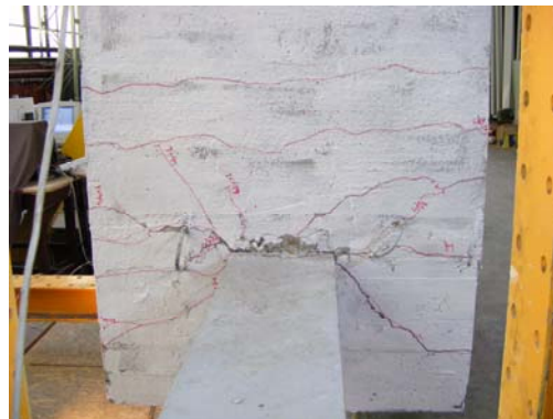
Fig. A.22. Concrete cracking at the beam-to-column joint under positive bending
