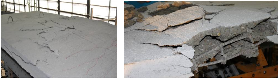
Fig. A.17. Local damage of the concrete slab over the link
