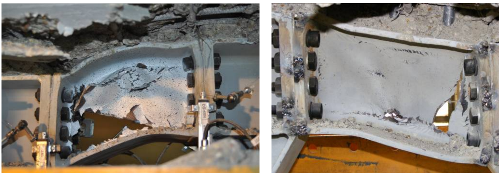
Fig. 3.48. Damage of the detachable link during the tests of EBF_Comp_LD1 and LD2
