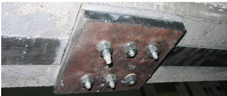
Figura 6.37. Detaliu ancoraj – grinda R-1S
