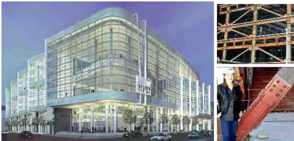
Fig. 2.34. Moscone West Convention Center with Pall Dampers in the braces, San Francisco, USA [26]
