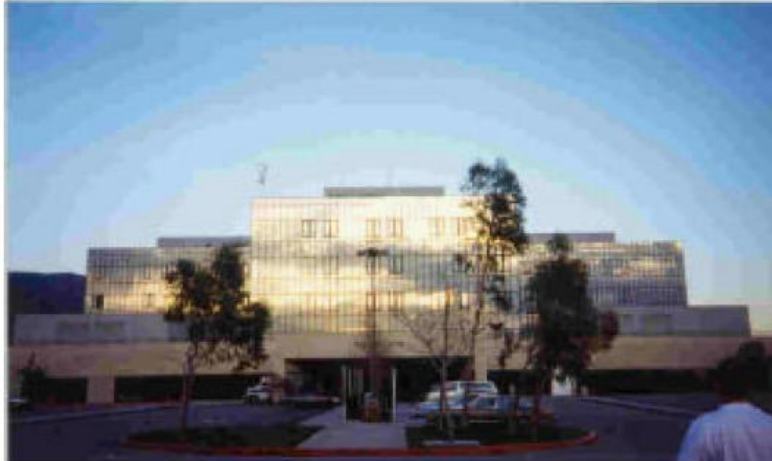
Fig. 2.13. Sylmar Hospital, Los Angeles, CA— 6 floors [16]
