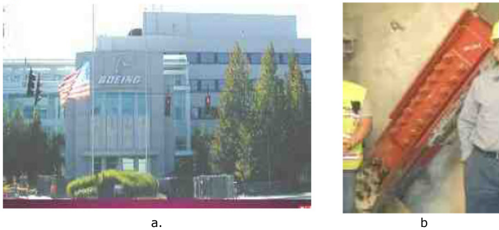
Fig. 2.35. Boeing Development Center, Cafeteria and Auditorium Buildings, Boeing Field, Seattle, WA, USA; a) general view of the building; b) Pall Friction Dampers used [26]
