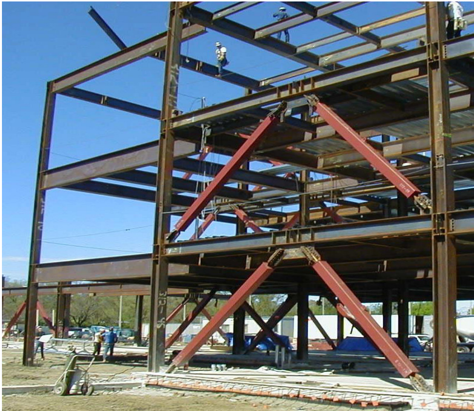
Fig. 2.22. UC Davis Plant and Environmental Science Facility [18]
