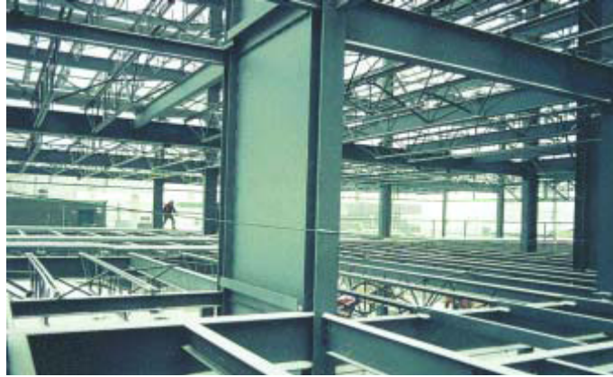
Fig. 2.11: Canam-Manac Headquarters Expansion, St. George, Quebec [1]
