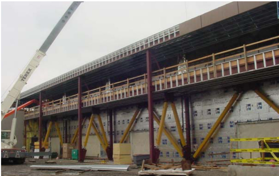
Fig. 2.21. Hewlett Packard building, Corvallis Campus, USA [19]
