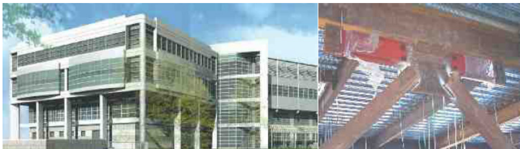
Fig. 2.36. Ambulatory Care Center, Sharp Memorial Hospital, San Diego, California, USA with Pall Friction Dampers in chevron bracing system [26]
