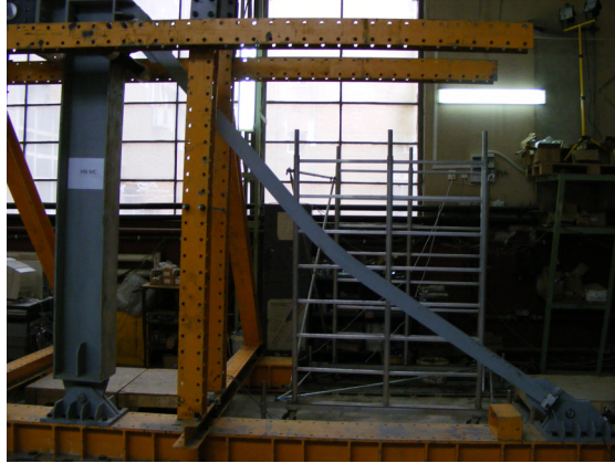
Fig. 3.35. Buckling of the HEA100 brace under monotonic compression load
