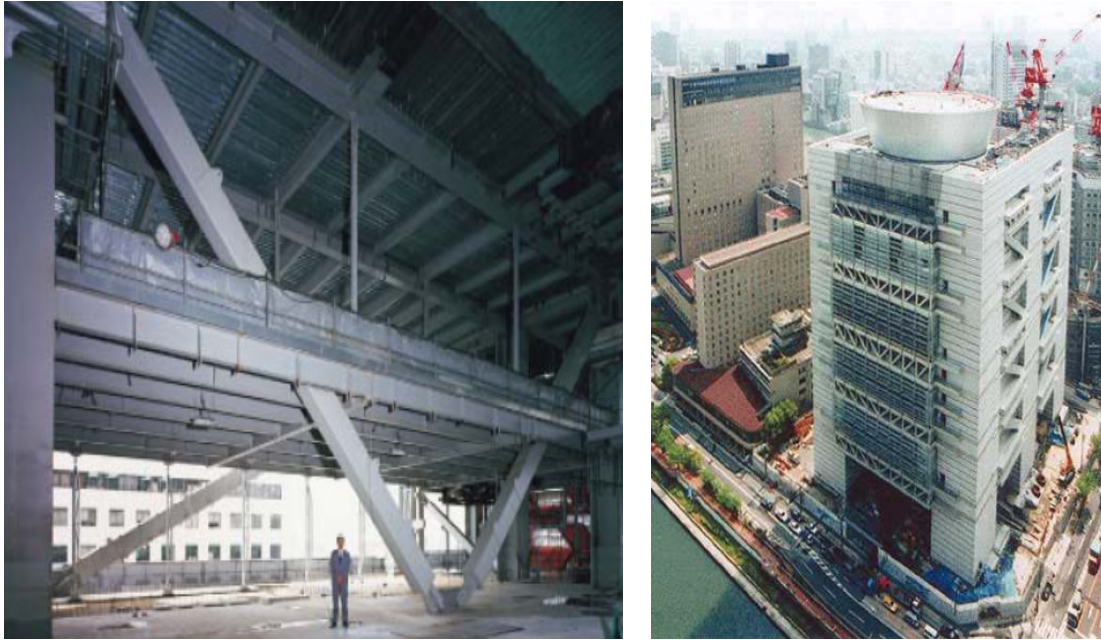
Fig. 2.20: Osaka International Convention Center (420 mil. US dollars project, 13+2 floors, 370 BRB's used) [19]
