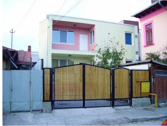
Fig.6.57 - C family house – completed house.
