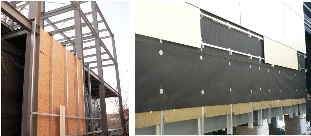
Fig.6.48 - Envelope during erection
