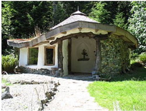
Fig. 3.54 - An example of a modern, Pacific Northwest-style cob home
