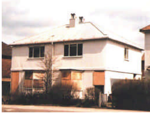
Fig. 4.25 Telford steel framed house -1920s- steel clad systems
