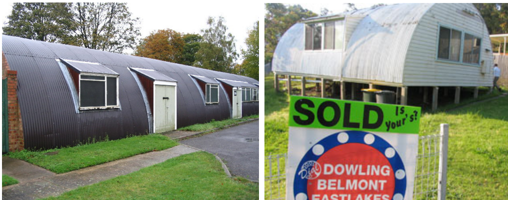
Fig. 4.22 – The Nissen hut adapted into a prefabricated house
