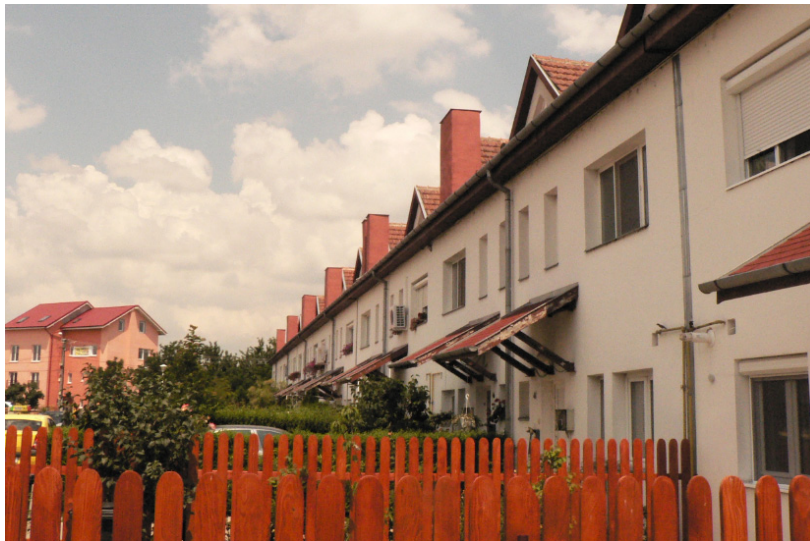
ANL ( National Housing Agency) Row Housing Development Timisoara
