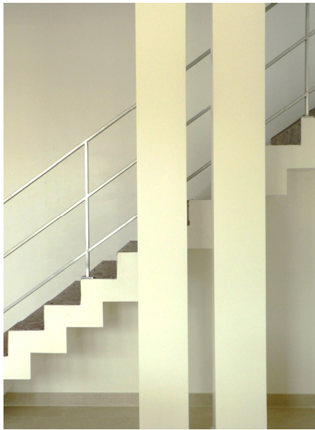
Fig. 6.34 – House P, stair case view
