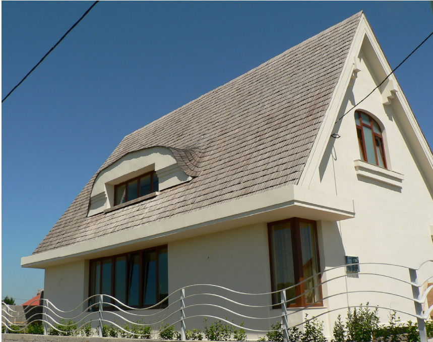
Fig. 6.17 – DM House, Timisoara, 2008- M. Mutiu, arch., View
