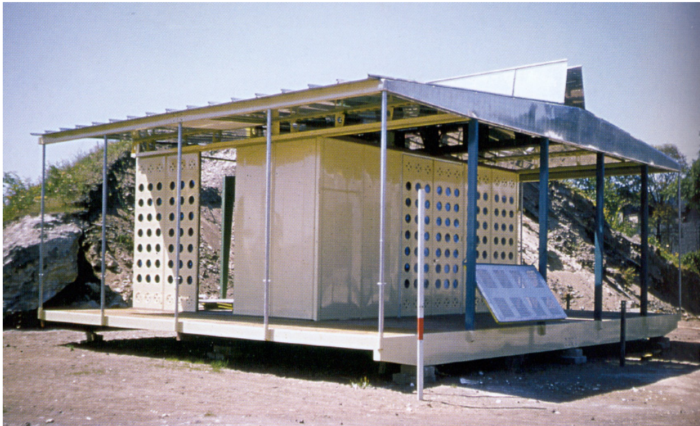
Fig. 4.56 Jean Prouvé –Maison Tropicale, Brazzaville, Congo, 1949 Steel Prefabricated Frames
