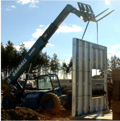
Fig. 5.14. Factory prefabricated wall
