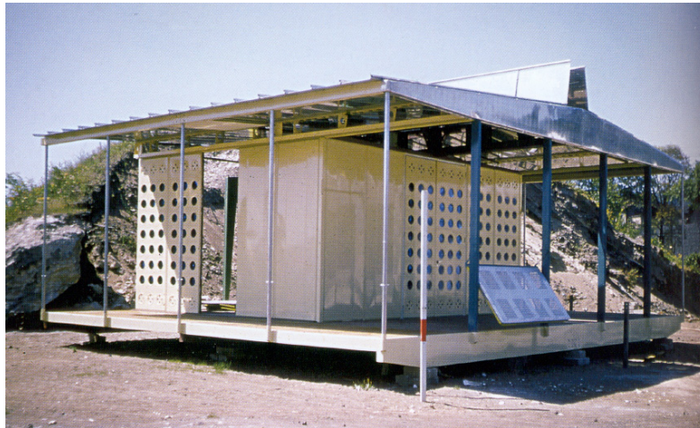
Fig. 4.17 - Jean Prouvé –Maison Tropicale, Brazzaville, Congo, 1949 Steel Prefabricated Frames
