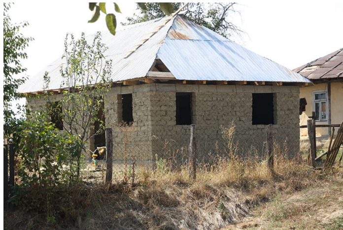
Fig. 3.51 - Romanian adobe house during construction
