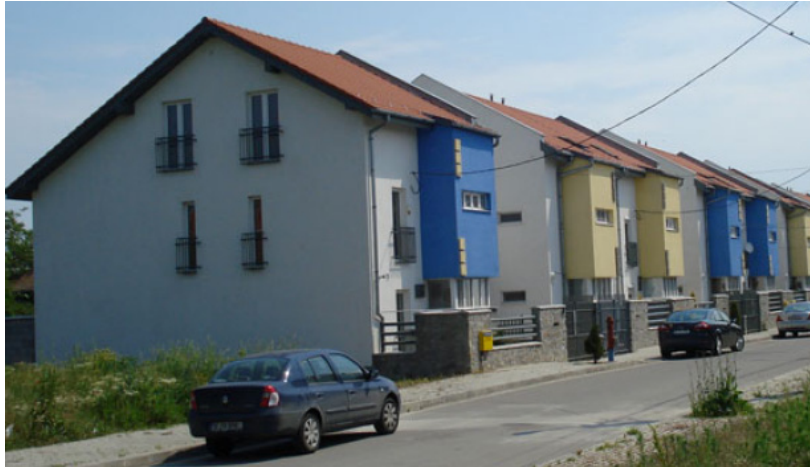
ANL ( National Housing Agency) Row Housing Development
