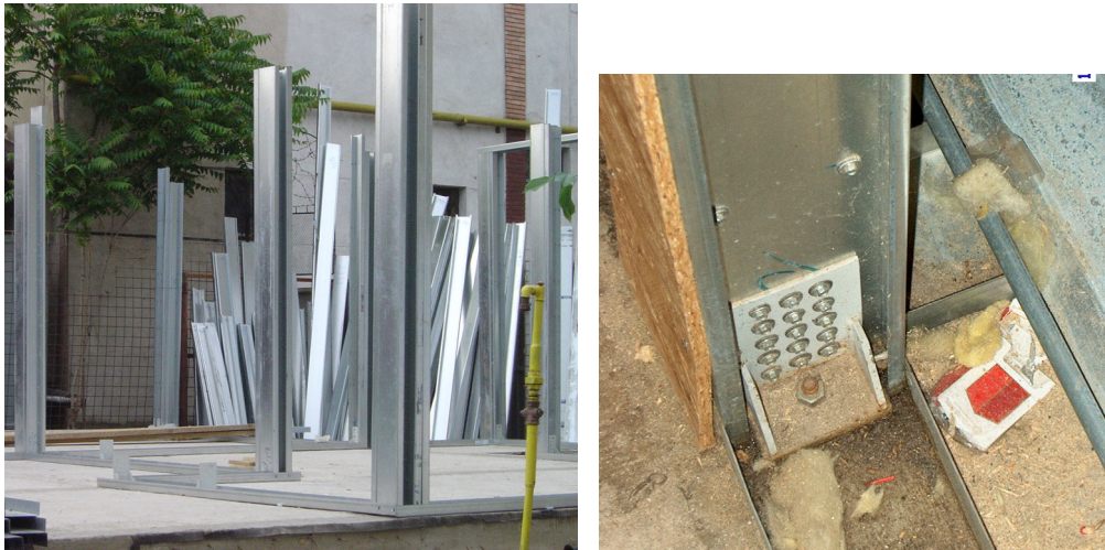
Fig. 5.37. Example of wall corner and hold down anchor realized in C. House
