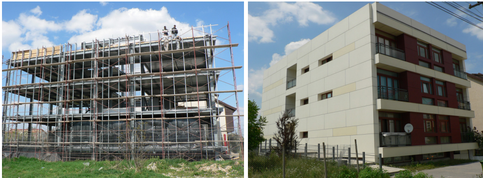
Fig.6.46 - Structure during erection and final view of the erected building
