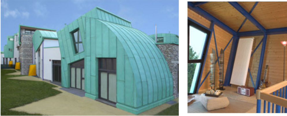
Fig. 4.28 The Ruginello row houses Roccatelier Associatti
