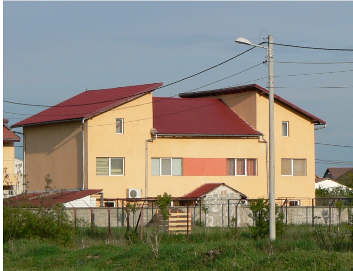
Fig. 3.4 House near Timisoara
