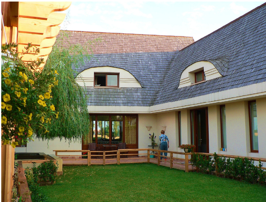
Fig. 6.18 – DM House, Timisoara, 2008- M. Mutiu, arch., Courtyard view
