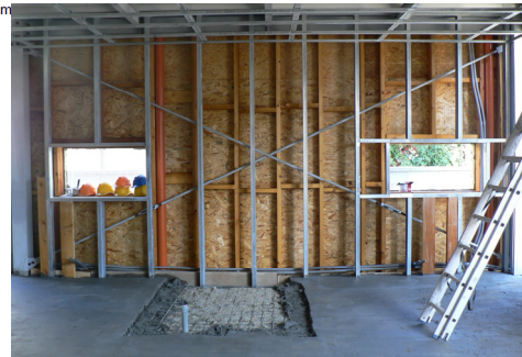
Fig. 6.29 – House P, wall assembly
