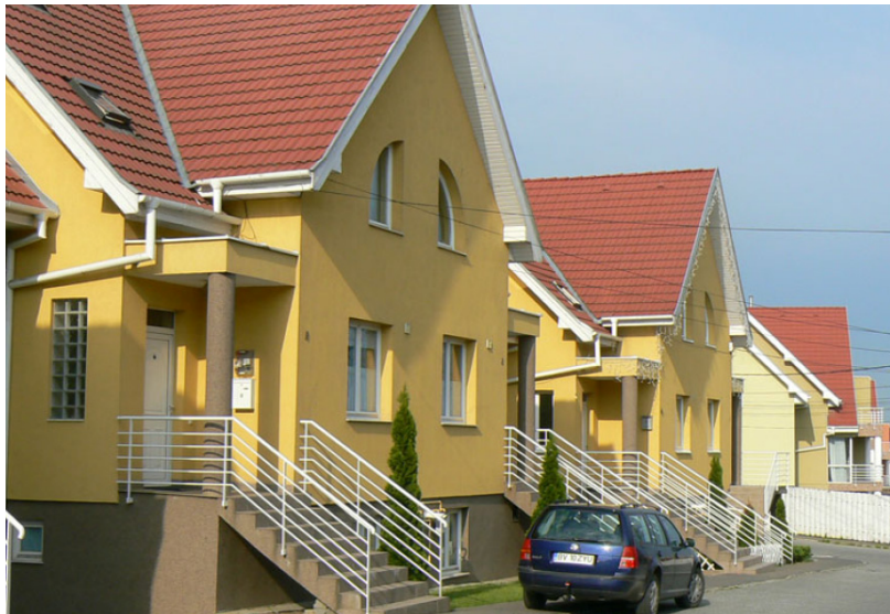
ANL (National Housing Agency) Row Housing Development
