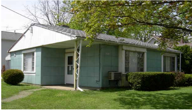
Fig. 4.24 - Lustron Corporation-family home, USA, 1948, prefabricated, all-steel house
