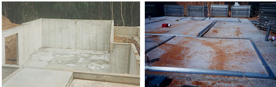
Fig. 5.18. Typical foundation systems [28]
