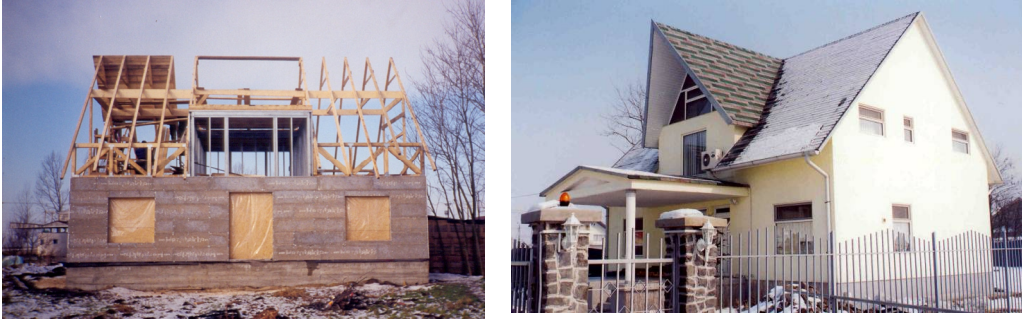
Fig. 6.6 - Skeleton of the structure and completed house.
