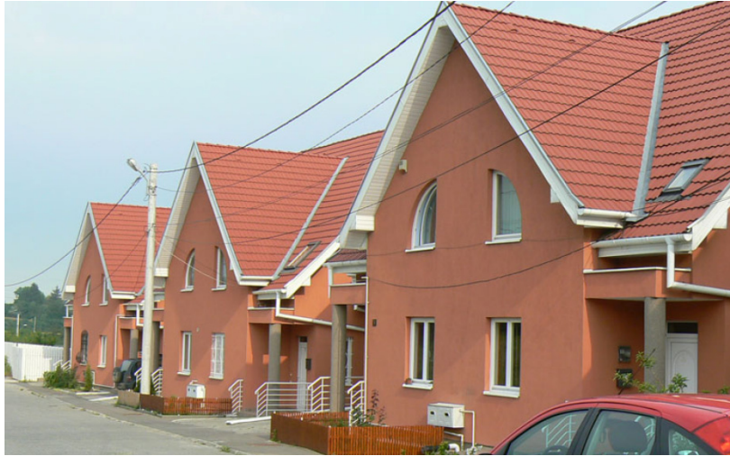
ANL ( National Housing Agency) Row Housing Development
