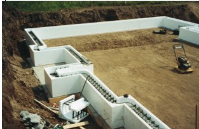
Fig. 3.57 - Insulated Concrete Forms Home
