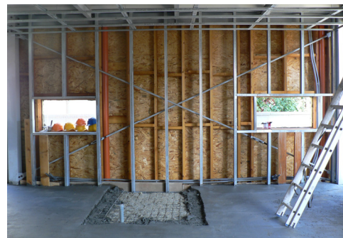
P. House Mixed Steel-Wood Envelope System
