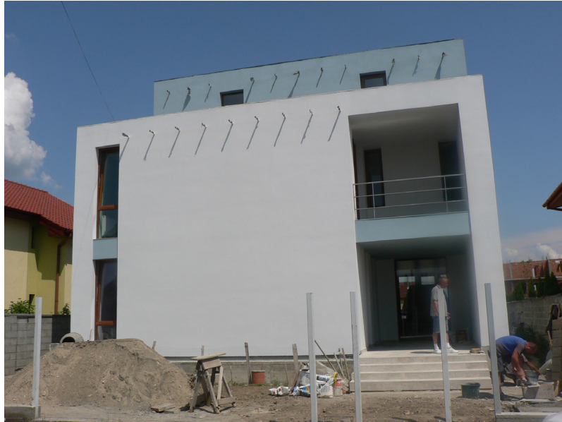
Fig. 4.54 M. Mutiu, P. House, Timisoara, 2010 – front view
