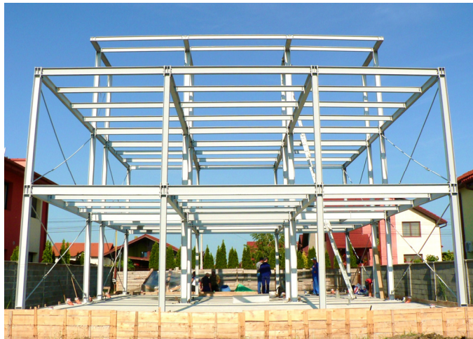
Fig. 6.27 – House P, Steel Frame view
