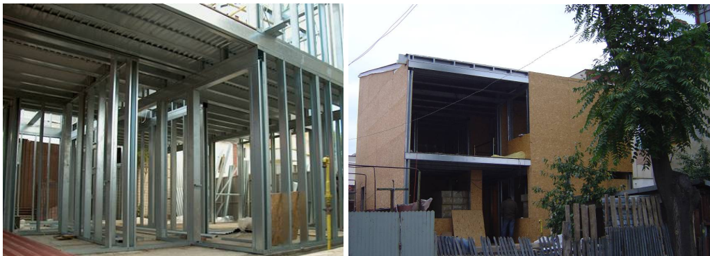
(a) the finished steel skeleton
