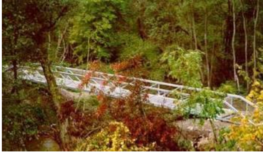
Fig. 2. 19. Aluminium trough bridge - Selzbach
