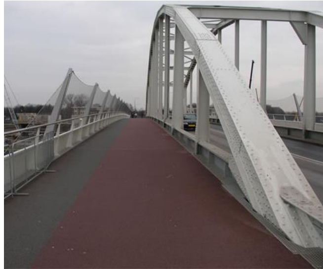
Fig. 2. 28. Bridge over Amsterdam-Rhine canal
