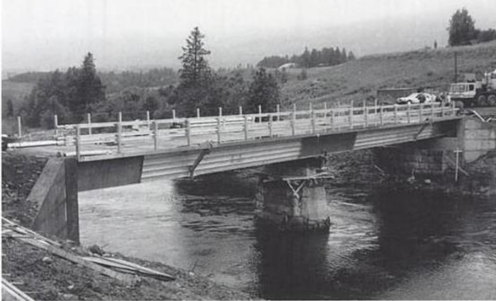
Fig. 2. 17. The Forsmo river aluminium road bridge (courtesy of Hydro Aluminium Structures)
