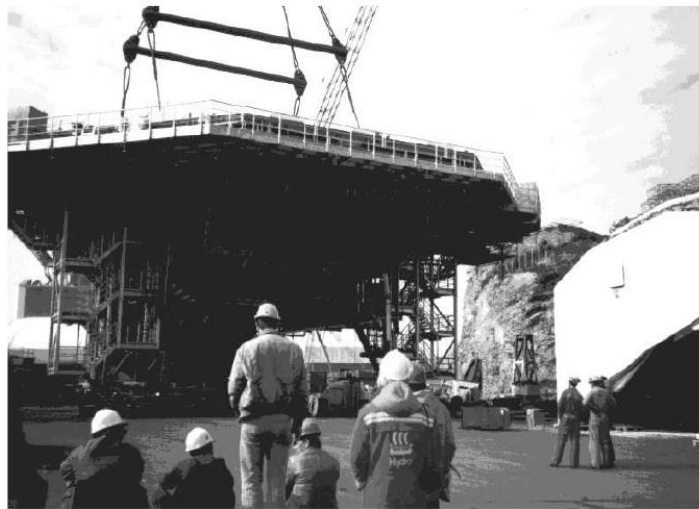
Fig. 2. 8. Offshore Aluminium Helimodule (Helideck, Helihangar, Stairtowers and support structure) – built in 1986
