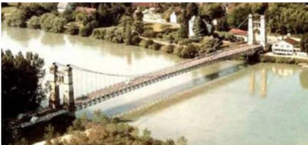
Fig. 2. 16. Lyon Groslee bridge (France)
