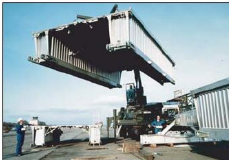
Fig. 2. 24. The German military bridge: erection phase
